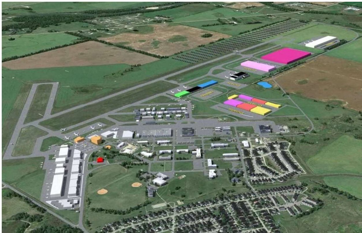
Figure 7. Satellite view of Edmonton International Airport (YEG)
